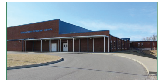
Morgantown Elementary School: Built 1972 ENERGY STAR® Rating 87
