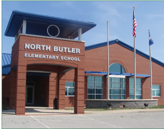
North Butler Elementary: Built 2005 ENERGY STAR® Rating 86
