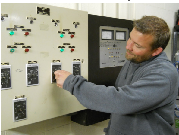
Billy Bramblett, Owen Lower Elementary School with older control system.
