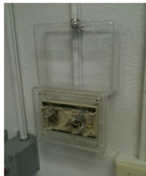
Broken thermostat set for heating & cooling at 72 degrees
